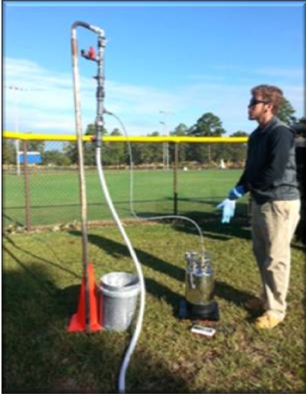
Typical injection point set-up is used during remedy augmentation on site SS028.
