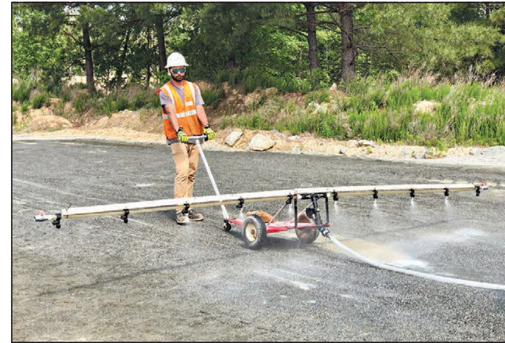
Kenley McAdams, from bioMASON, applies a feeding to the bacteria to harden the surface of the Project Medusa 2,500 square foot prototype in Durham, North Carolina.
