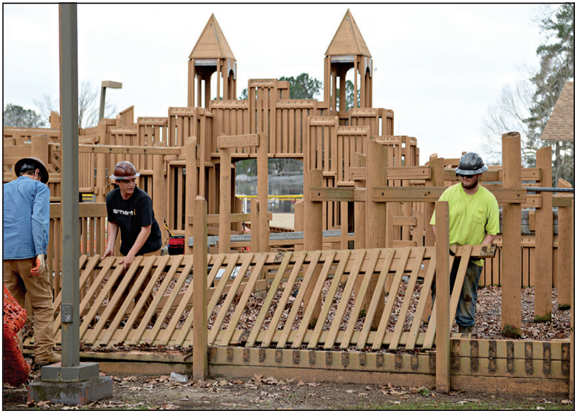
U.S. Air Force photo by Airman Hannah Bean Construction workers disassemble pieces of Freedom Park during demolition Feb. 6, 2019, on Columbus Air force Base, Mississippi. The Freedom Park playground was built in 1996, a time when playgrounds were typically constructed with wooden materials.
