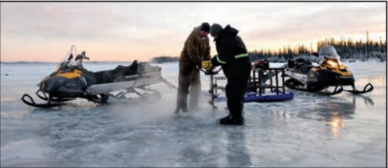
Senior Airmen Tyler Dray and Jerry Mitchell use an ice auger Nov. 20, 2014, while constructing an ice bridge in Fairbanks, Alaska. The bridge must be constructed every other year to provide access to the $20 million range complex used to train pilots from around the world during Red Flag-Alaska exercises. Dray is a range maintenance structures journeyman and Mitchell is a heavy equipment operator with the 354th Civil Engineer Squadron on Eielson Air Force Base, Alaska.
