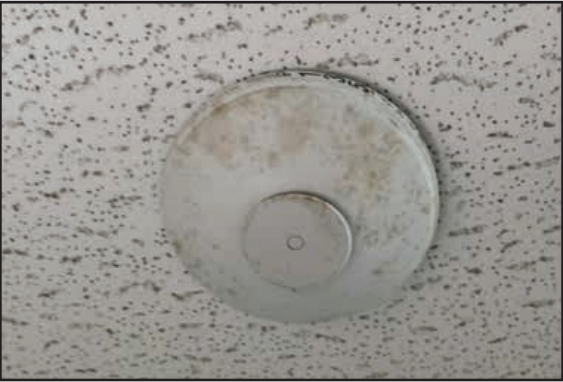
Figure 2: Smoke detector — Mold is visible here and hidden on the tile
