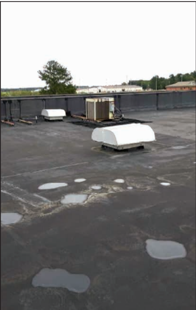
Courtesy photo The prior roof was replaced because of water leaking through the roof into the Base Exchange. CYE Enterprises was awarded a contract to replace the roof.
